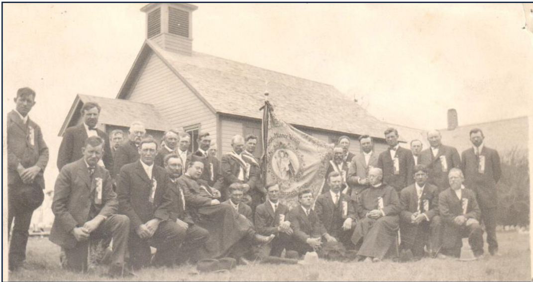
St. Joseph's Verein, Nazareth, Texas, 1913. Attached to the back of the church building may be seen the roof of the room built in 1903 which was used as the church until the front part was added in 1908 or 1909. The roof and chimney extending to the right of this one room are those of the section added as living quarters for the priest.
